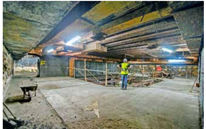
The top floor of the R4 operations room in 2001 showing the damage caused by the fire. Before the fire the well has been floored over with timber. Photo Nick Catford
